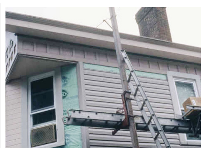
FIGURE 12.6 Installation of replacement siding.
