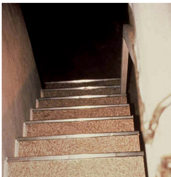
FIGURE 18.6 Enclosure of stairs in this manner is generally not appropriate in a historic property.
