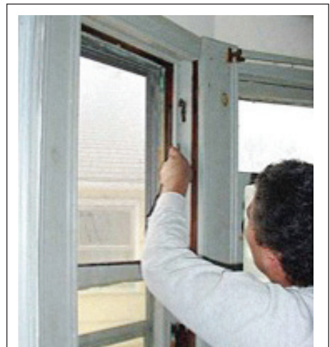
FIGURE 11.6 Remove parting Aboard.
