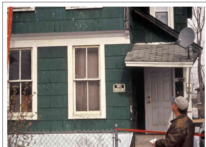
FIGURE 3.1 Assessing the physical condition of a property.
