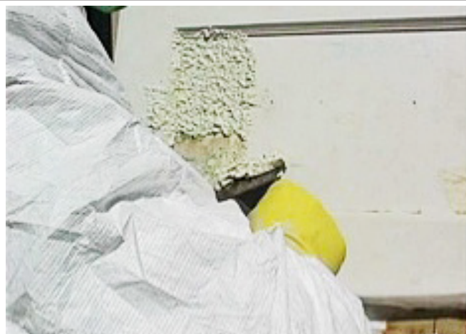
FIGURE 12.20 Workers should wear protective clothing when using chemicals.
