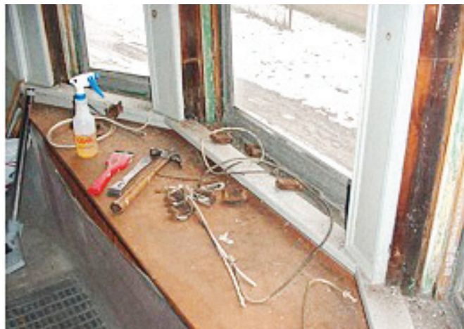
FIGURE 11.9 Window after removal of sash weights.
