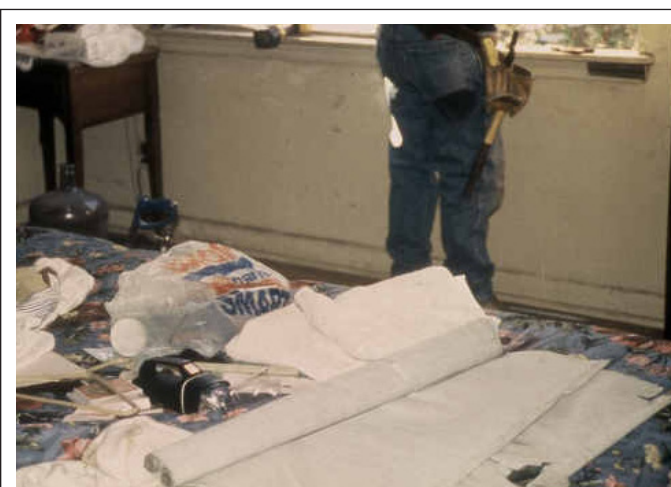
FIGURE 4.3 This worksite was not properly prepared for lead-disturbing work by removing the occupant's belongings.
