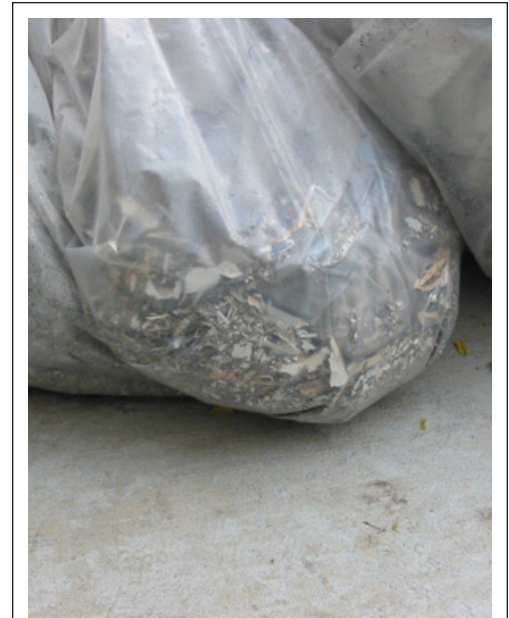
FIGURE 10.4 Paint chips should be double-bagged and seams sealed.
