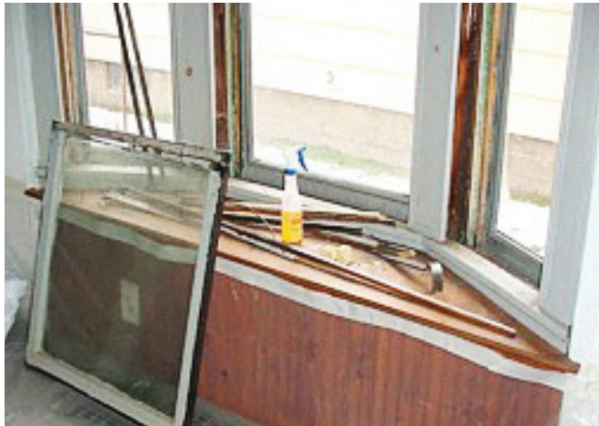
FIGURE 11.7 Remove the bottom sash, sash weights and stops.
